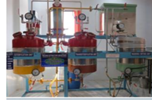
Bio -Diesel Plant
